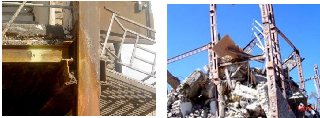
Fig. 2. Brittle saddle connections failure - total collapse examples in Bam earthquake (Mw. 6.5, 2003) [9]
