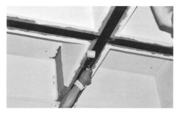
Fig. 4-1: Flexural strengthening of RC beams with CFRP strips.
