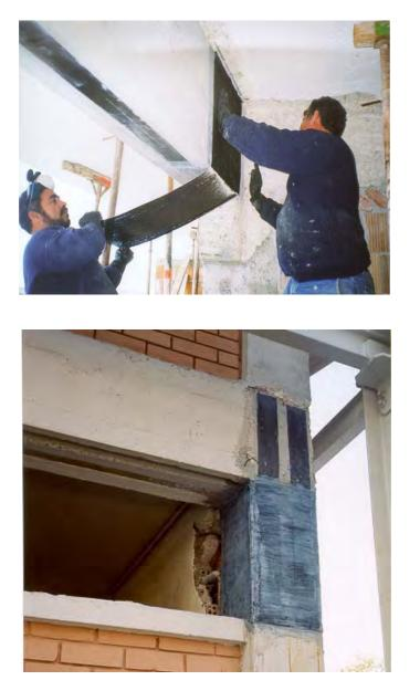
Fig. 5-3: Shear strengthening of: (a) beam end; (b) short column.
