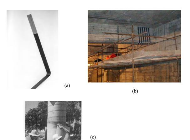
Fig. 2-8: Examples of prefab shapes for strengthening. (a) angle, (b) application of angles, (c) shell.
