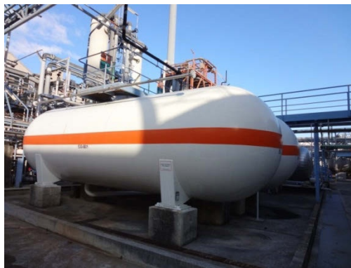
89 90 Figure 1: Horizontal cylindrical reservoirs resting on four legs system support
