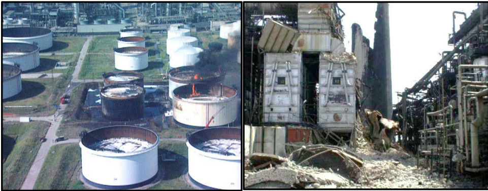
77 78 Figure 1: Damaged tanks at tank farm (left) and collapsed stack at TÜPRAŞ Refinery
