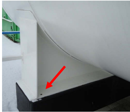
Figure 3: Horizontal cylindrical reservoirs resting on saddles
