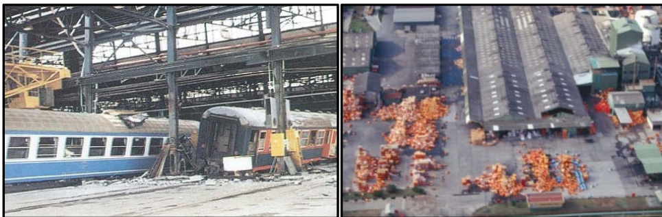
102 Figure 4: Damaged steel structure at Adapazari rail car factory (left) and losses of open 103 stored materials
