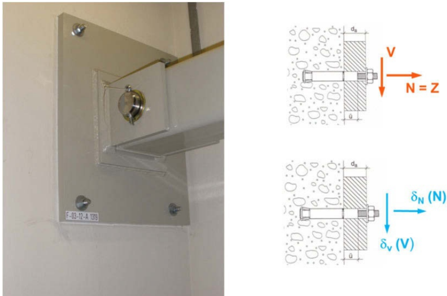
Figure 1: Anchoring with metal anchors (acting forces N and V with corresponding displacements \delta_N and \delta_V )
