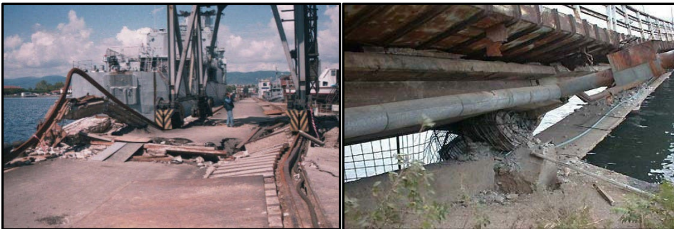
178 Figure 7: Damage at navy port in Gölcük (left) and failed column at SEKA port
