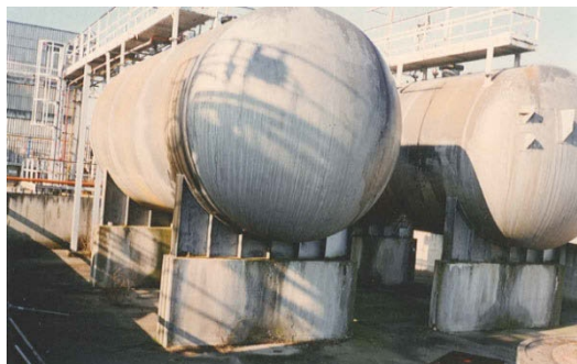
91 92 Figure 2: Horizontal cylindrical reservoirs resting on saddles of support
