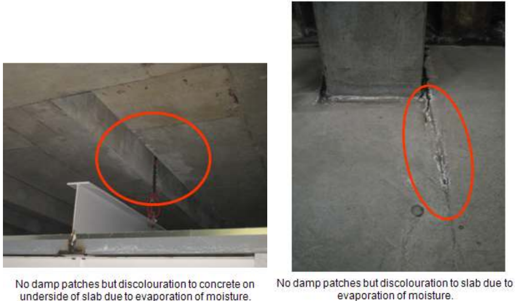
Figure 5: Typical conditions within a Grade 2 Basement.
