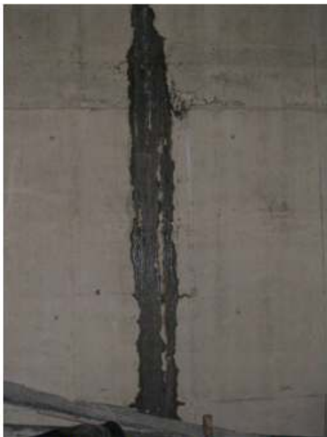
Leak through joints in concrete wall. Water is 'running' therefore exceeds 'some seepage' criterion.
