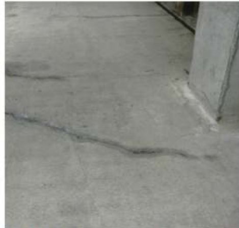
Grade 1 internal environment. Some seepage and beading through cracks but water not flowing.
