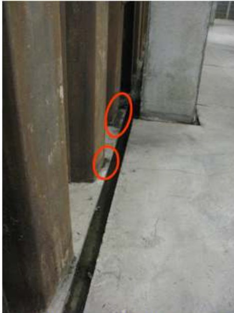
Grade 1 internal environment. Damp patches on slab. Traces of water in channel on floor.
