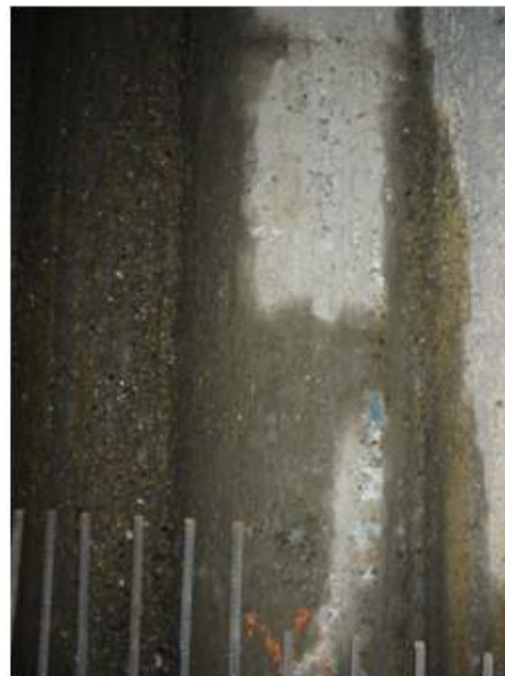
Leak through joints in secant pile wall. Water is 'running' and damp patches exceed 10% of wall face.
