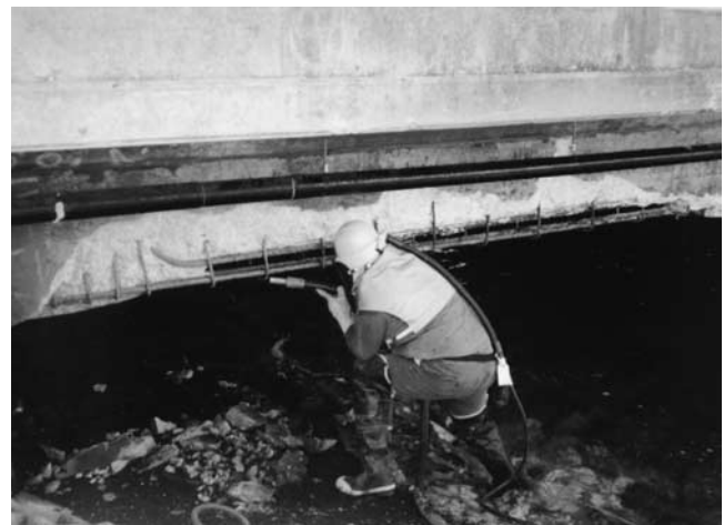
Figure 3.2. Sandblasting of corroded steel.
