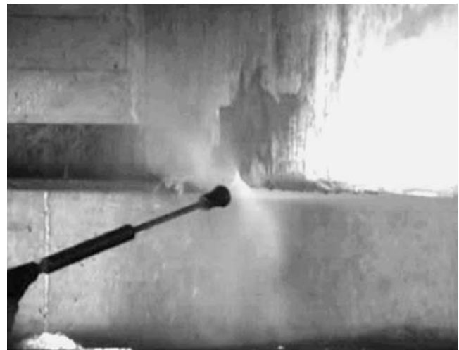
Figure 3.6. Pressure washing of concrete.
