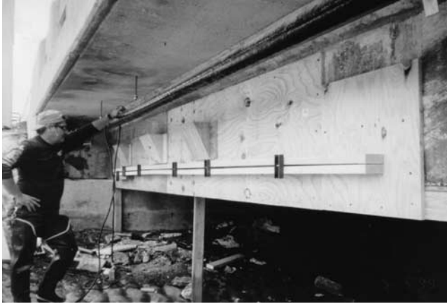
Figure 3.4. Forming concrete section.
