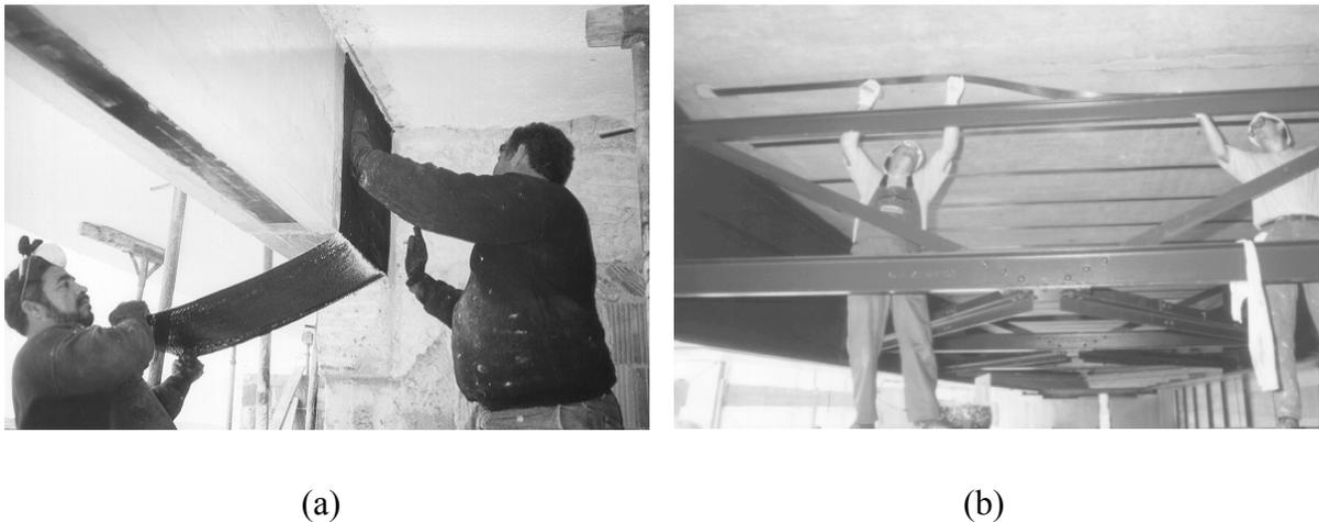
Fig. 2-2: (a) Hand lay-up of CFRP sheets or fabrics. (b) Application of prefabricated strips.
