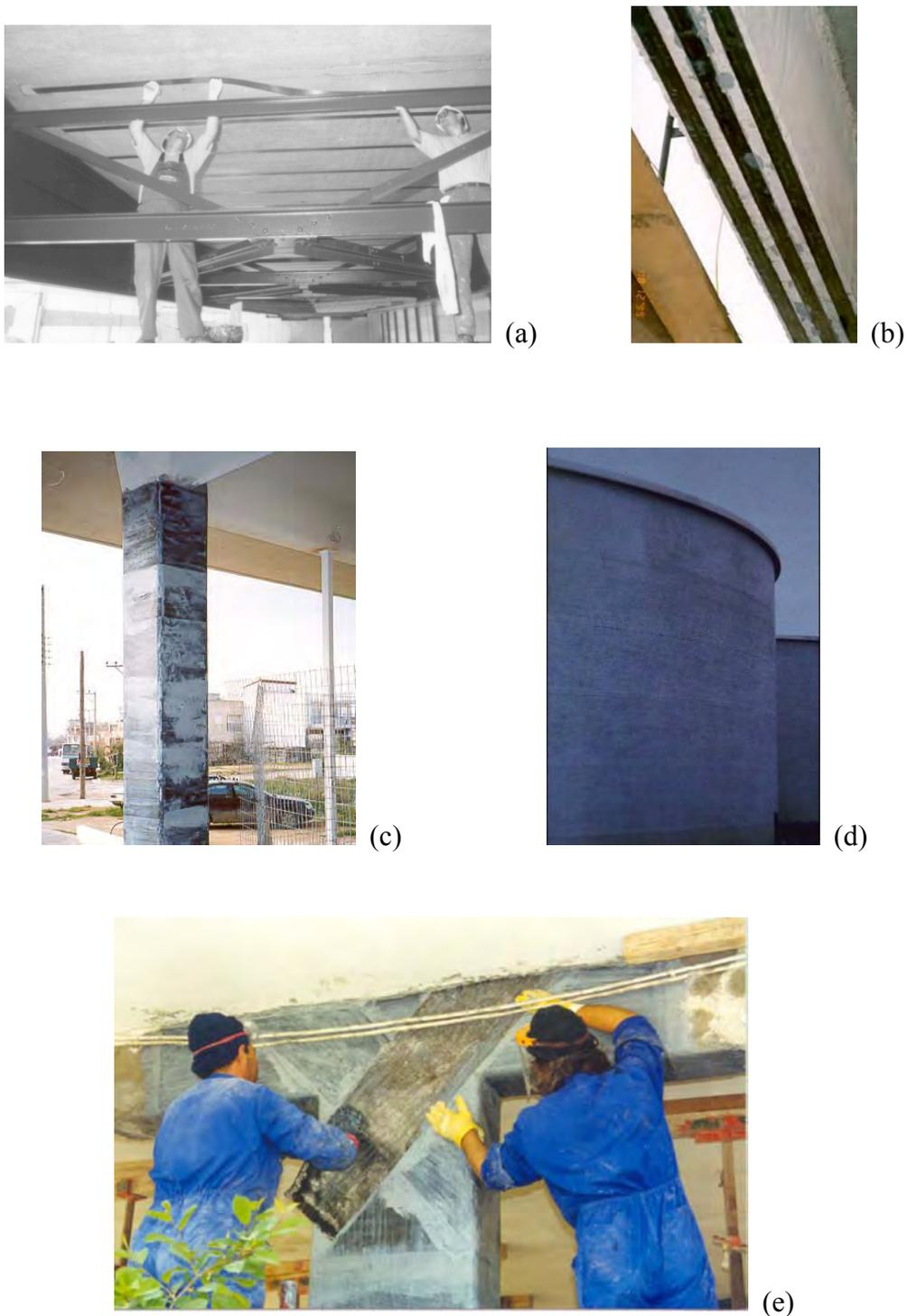
*Fig. 1-2: Typical FRP applications as strengthening materials of RC structures: (a) flexural strengthening of slab; (b) flexural strengthening of beam; (c) shear strengthening and confinement of column; (d) wrapping of concrete tank; (e) shear strengthening of beam-column joint.*
