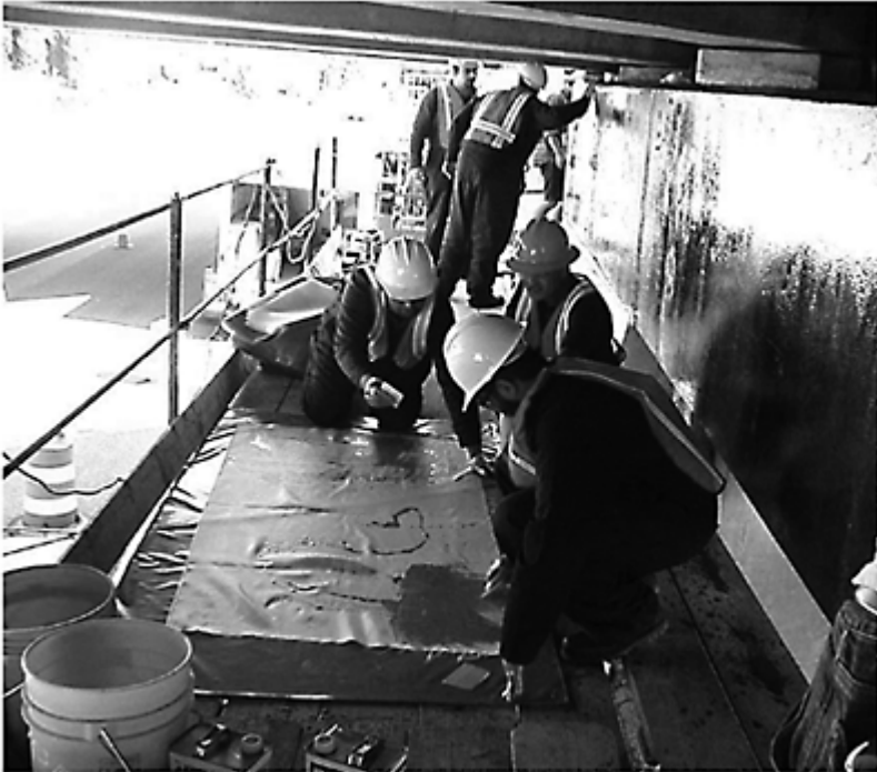
Figure 8.1 Retrofitting with composite material jackets: (a) hand lay-up of fiber-glass with epoxy by the authors; (b) machine winding of carbon fiber and epoxy (Source: XXsys Technologies, Inc., 1997).
