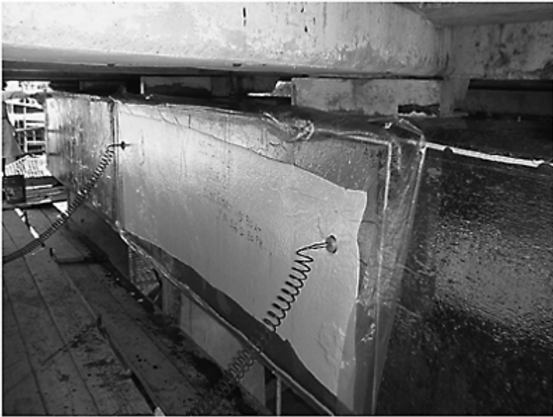
Figure 1.1 Vacuum bagging technique for rehabilitation of reinforced concrete bridge pier.
